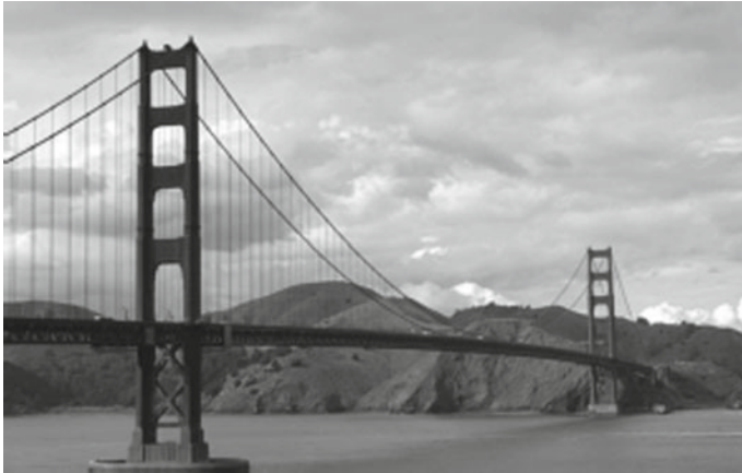
Fig. 5.1 Golden gate bridge (Wikipedia)
