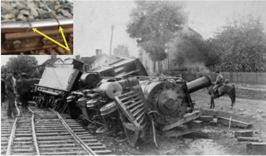
Fig. 7.11 Fracture of train wreck due to metal fatigue failure of rail from Wikipedia
